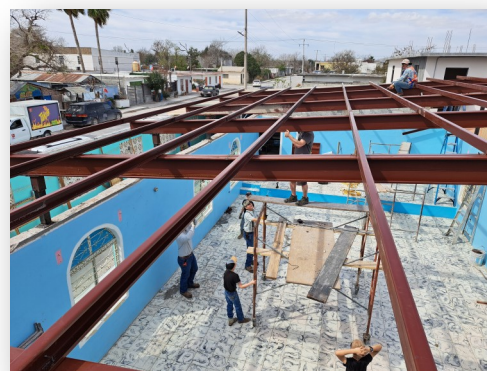
Progreso work team building new roof
