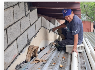
Pastor Moises, the pastor of the church, laying block
