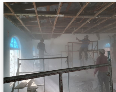
Demolition work to remove the old ceiling and roof
