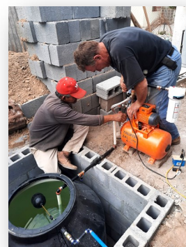
Perry and Teno building a new water system
