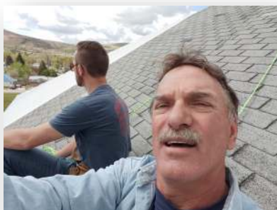
Pastor James Peterson and myself starting to put on the steel roof
